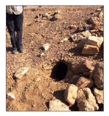
While it is not known if these burrows are present at the time of the embankment being breached they certainly need to be removed and the void repaired during any rehabilitation. Also the community must be informed of the dangers of allowing animals to establish burrows in the embankment.
